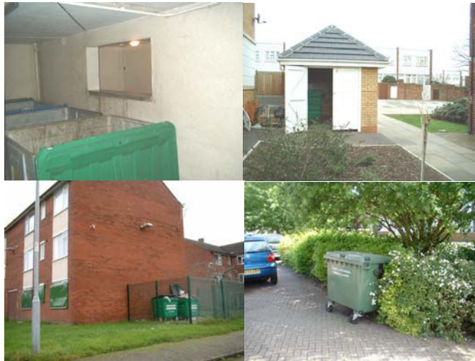
Bring Refuse Systems for Blocks of Flats: Top left: internal bin room reached by hatch, ground floor 12 storey block Brighton. Top right: External bin shed serving four-storey blocks of flats Redbridge. Bottom left: Fenced open air bin compound at side of three-storey block Crewe & Nantwich. Bottom right: Informal bin area in car park for block of flats in South Bedfordshire.
